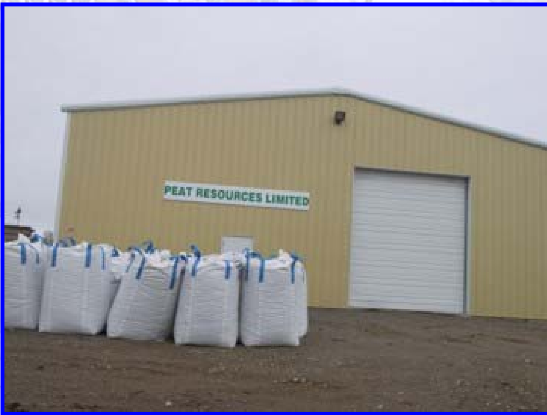
Peat Resources' Pilot Plant in Stephenville
