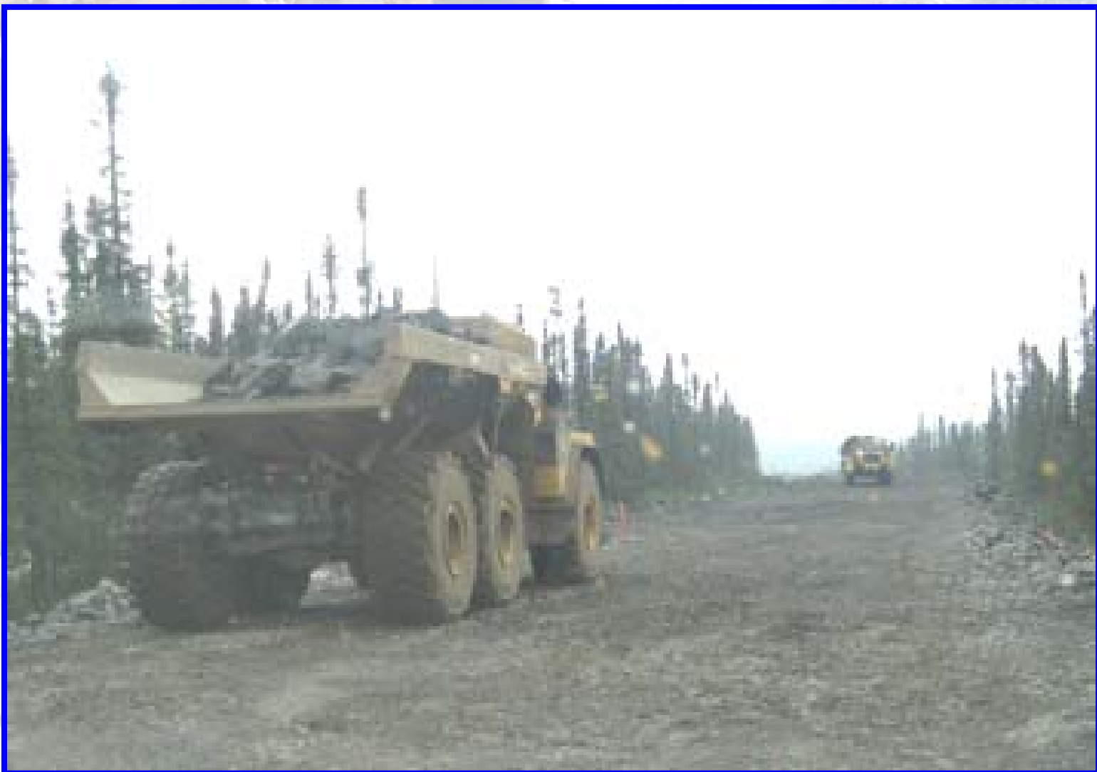
Preparation of rough grade for the overland conveyor
