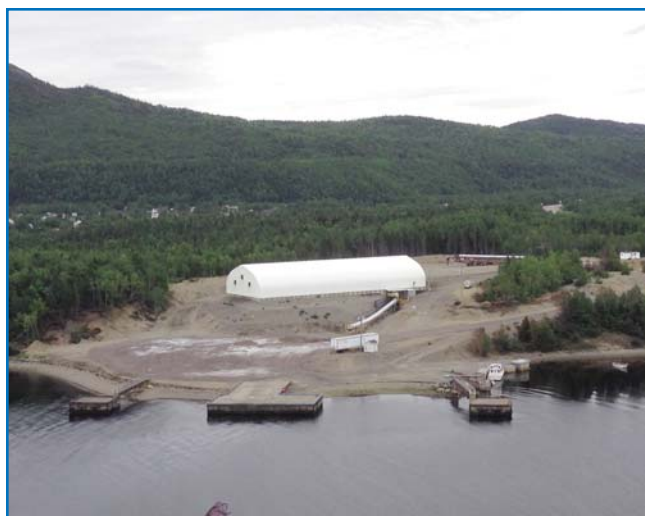
Rambler's concentrate storage shed at Goodyear's Cove
