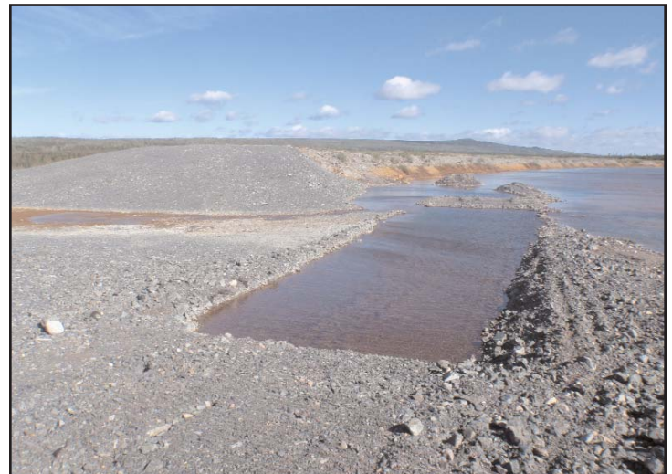
Gullbridge Dam Breach Area After Repair, 2013
