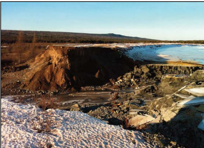
Gullbridge Dam Breach, 2012
