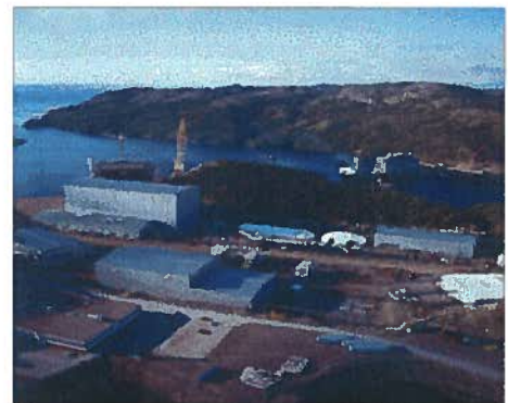
Topsides Fabrication and Assembly Area
