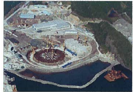
Drydock Construction and Fabrication Site
